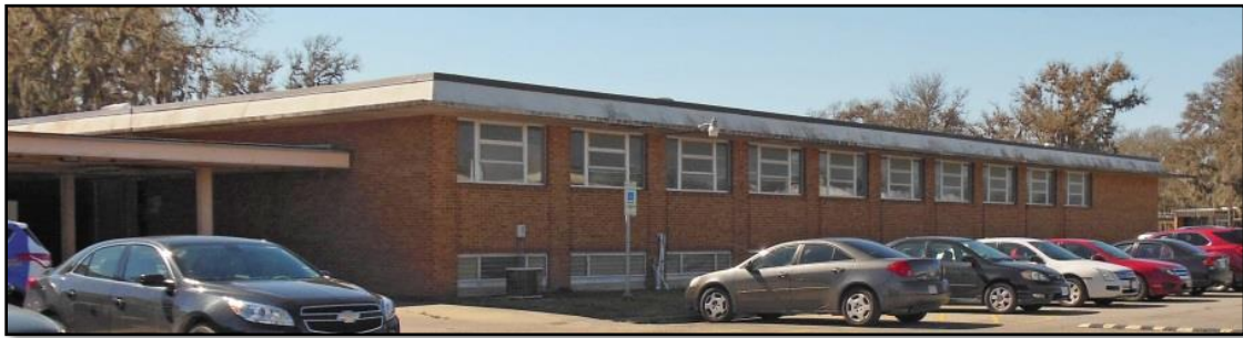
Central Laundry, which services three SSLCs
