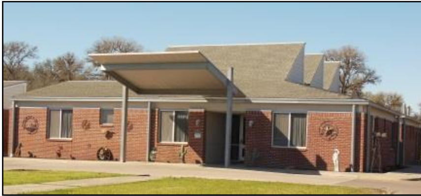
One of five residential cottages
